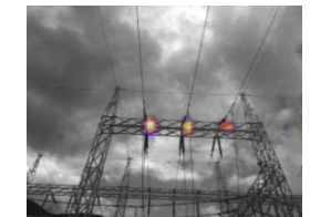
Transmission tower maintenance
