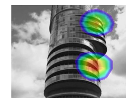
Building maintenance (Abnormal Noise Source)
