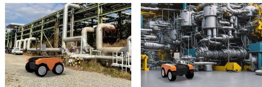
Driving robot-based Industrial Facility Diagnosis System
